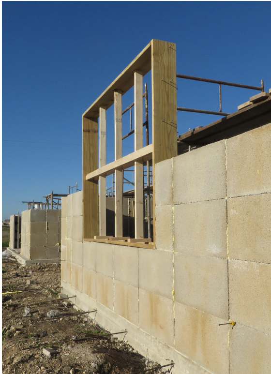
Figure 12: Stay-in-place wooden window buck
