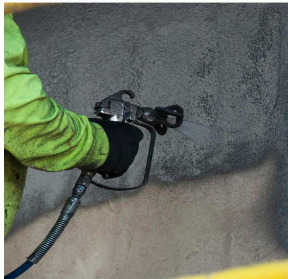
Figure 18: Application of air and moisture barrier
