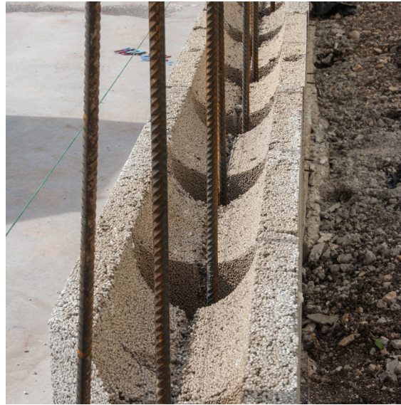
Figure 2: Laying first course of Bautex Block
