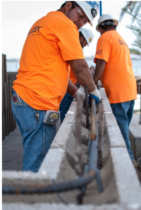
Figure 5: Placing horizontal reinforcing steel
