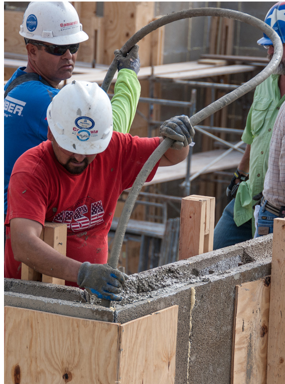
Figure 16d: Pencil vibrator on whip during wall pour.
