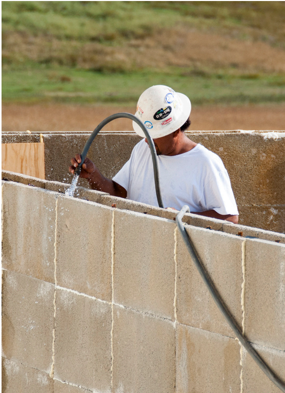
Figure 16a: Pre-wetting of forms prior to pour.
