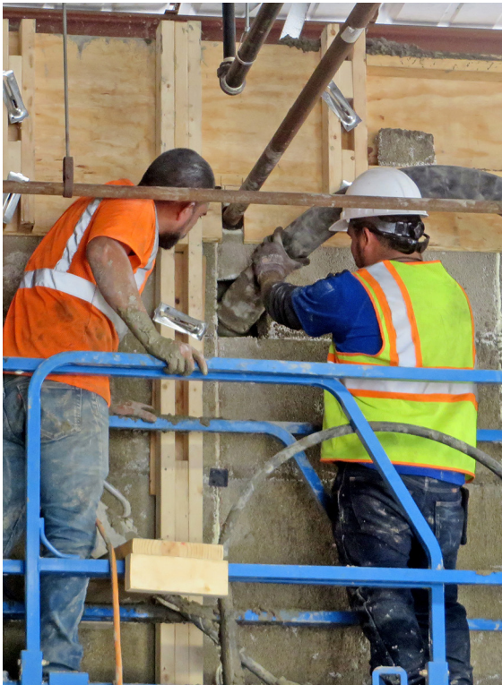
Figure 16c: Wall pour under existing structure.
