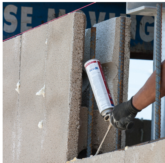
Figure 13: Bond beam cut out of Bautex Block
