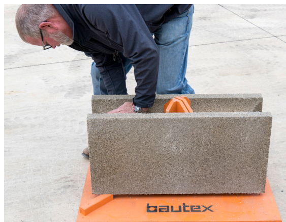
Figure 4: Simple and inexpensive 90° corner saw guide.
