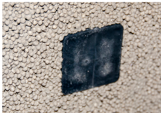
Figure 10: Bautex Wall Anchor installation
