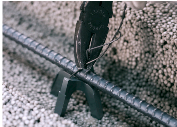
Figure 7: Tying reinforcement to rebar chair
