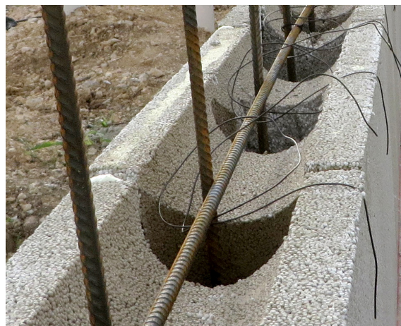
Figure 8: Wire loops for vertical reinforcement ties
