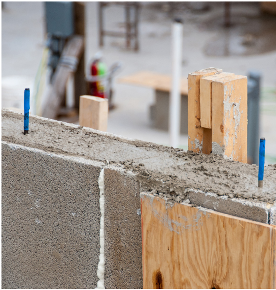
Figure 14: Wet-set J-bolts for wall top plate
